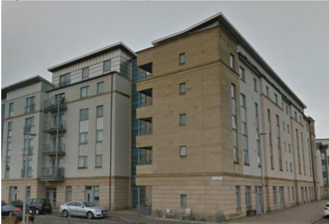
Image 11: Modern new build flat (2000s)
