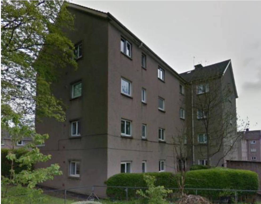
Image 7: Cavity built tenement flat (1950s)
