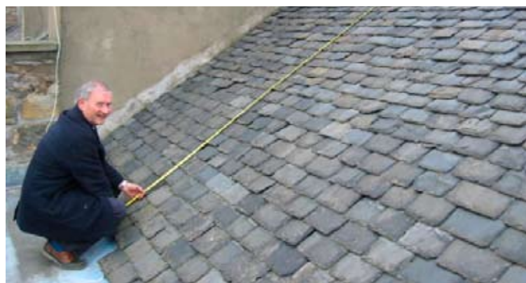
Measuring the roof for the solar panels. © Changeworks.
