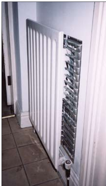
Radiator with reflective radiator panel
