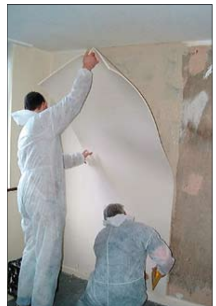
Insulation sheet applied to walls
