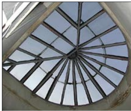
General view of ceiling to a close, showing rooflight
