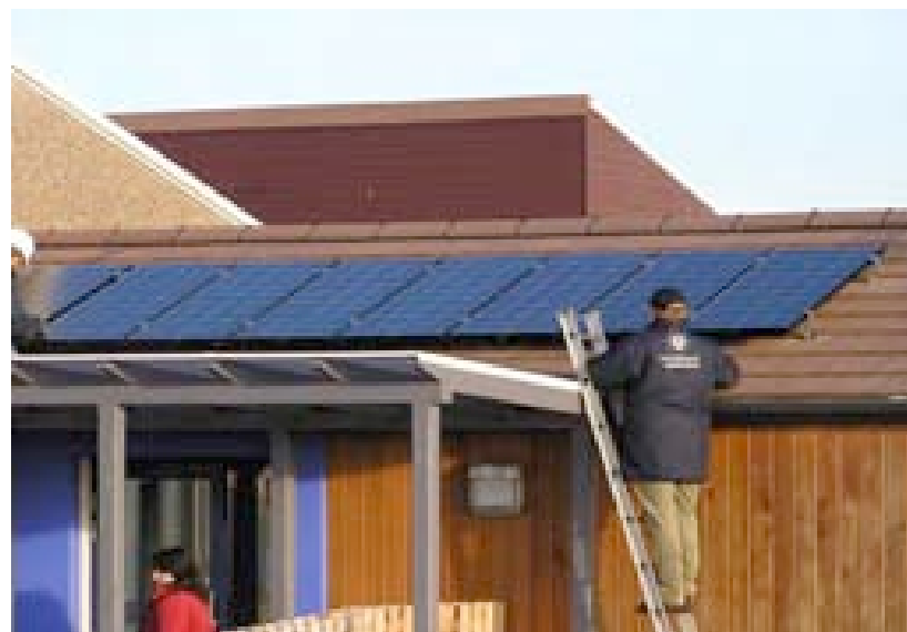
Gullane Primary School Under Construction
