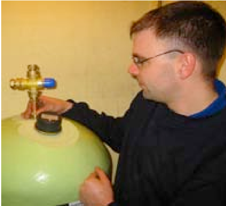
6. Mixer valves to control temperature.
